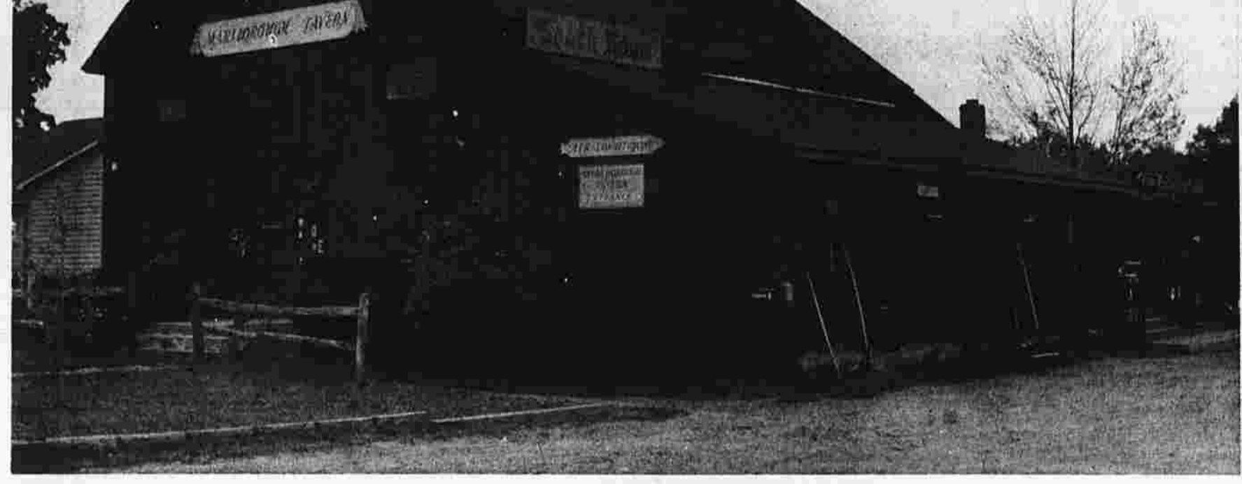
Historic Marlborough Tavern in Marlborough, Conn. (Photo by Floyd Larson)
